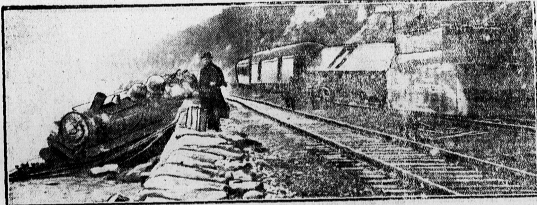
A number of passengers were injured when a slide of earth struck a train near Richmond Beach, Washington, recently. The locomotive was swept from the track and overturned
