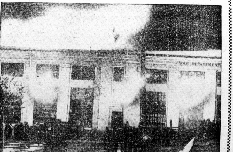
While 500 troops from Ft. Myer, Va., guard the ruins, federal authorities investigating the mysterious fire which swept three new wings of the War Department Building in Washington. Above, flames shoot from the structure at the height of the blaze. Important record files were in offices burned, one of which was Army Air Corps code room.
