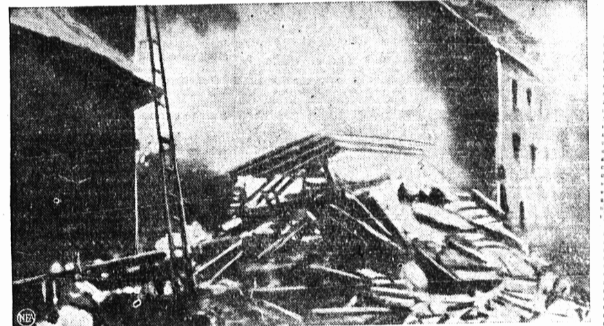
Smoldering ruins of shattered Helsinki apartment buildings and business houses were left in the wake of Soviet air raiders whose incendiary bombs fired large sectors of the Finnish capital.
