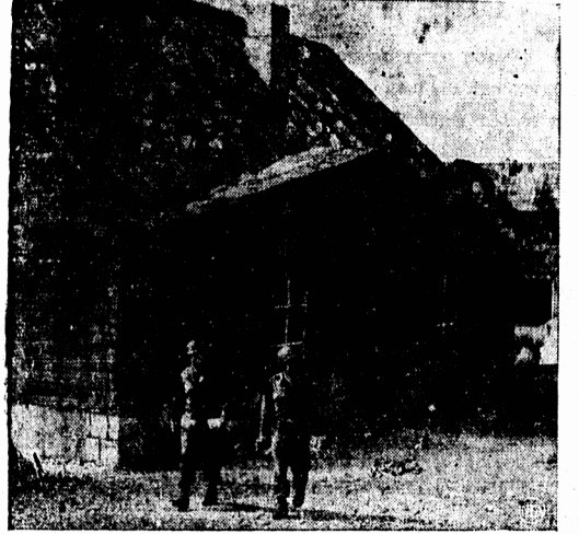
Very deceitful creatures, those Nazis. Photos above show two examples of elaborate camouflage found by tanks somewhere in France after Germans fled. Top photo shows what's apparently the stark skeleton of a bombed building. It is a complete fake, having been carefully constructed by Germans to fool Allied airmen into passing up the area. The "ruins" conceal large underground barracks. Also built to hide subterranean quarters was the "farmhouse" in bottom photo. It was painstakingly constructed of plywood and netting, elaborately painted for realistic effect.
