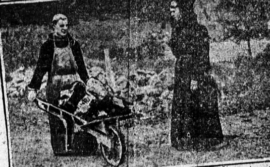
At work on the foundation of the abbey
