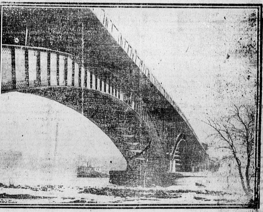
The above photograph of the Vehicular Peace bridge was taken from the Canadian shore, looking towards Buffalo. On the Canadian side, its terminal will be on the ground on which was fought the battle of Fort Erie, in the war of 1812. On the American side the terminal will be on land now occupied by the buildings of Fort Porter in Buffalo. This bridge will be open to traffic about the first of June. It is expected that the Prince of Wales and President Coolidge will formally open the bridge in August of this year.
