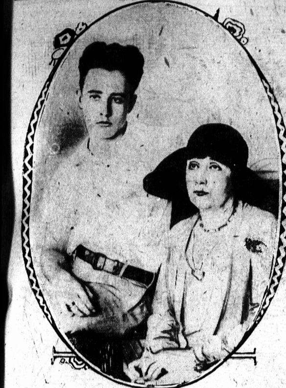
Above is Mrs. D. E. Chipps, widow of the slain lumberman, and her son, taken in the courtroom when Rev. J. Frank Norris was put on trial for murder. The trial has now been postponed until January.
