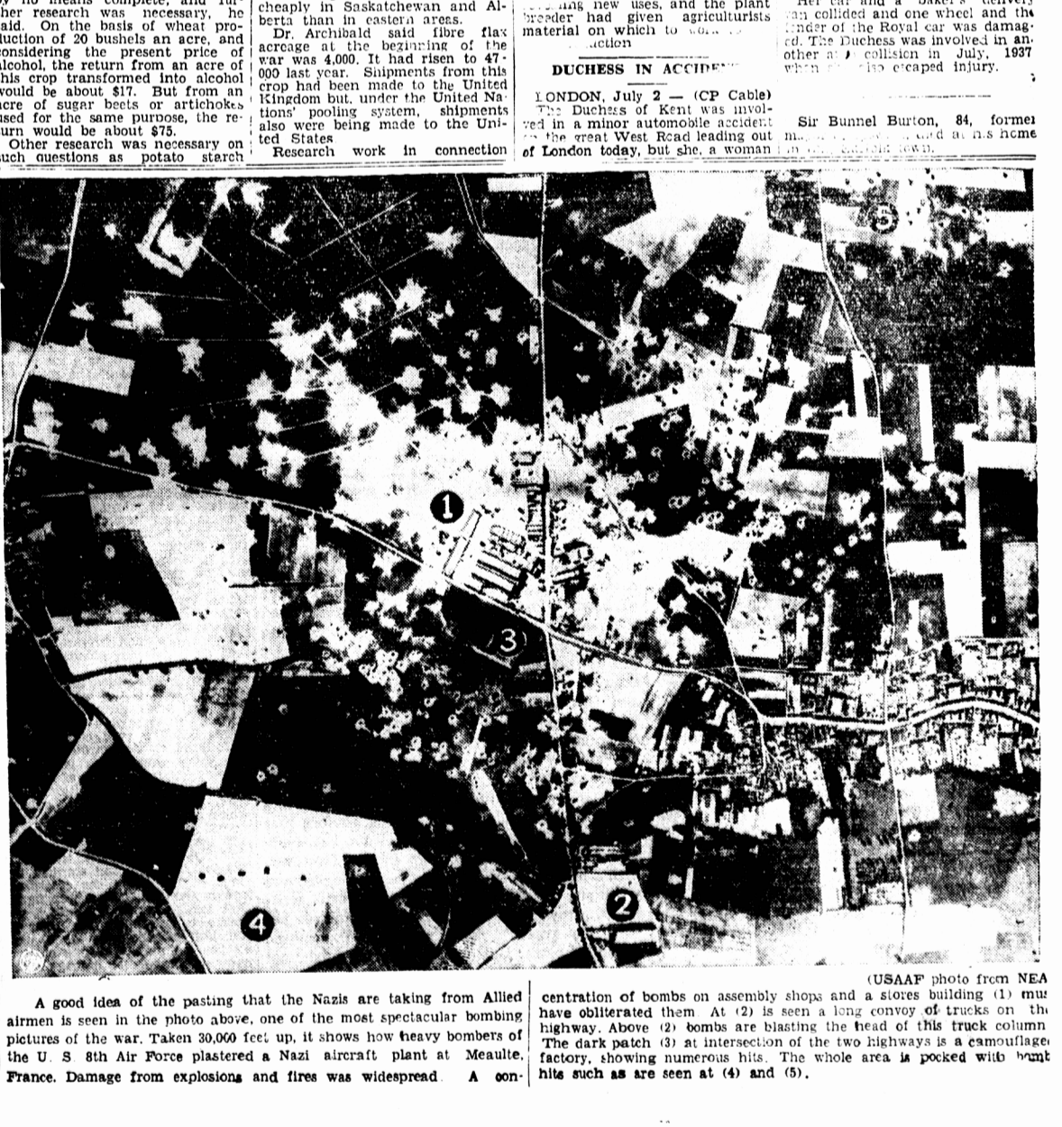
USAAF photo from NEA concentration of bombs on assembly shops and a stores building (1) must have obliterated them. At (2) is seen a long convoy of trucks on the highway. Above (2) bombs are blasting the head of this truck column. The dark patch (3) at intersection of the two highways is a camouflage factory, showing numerous hits. The whole area is pocked with burnt hills such as are seen at (4) and (5).
