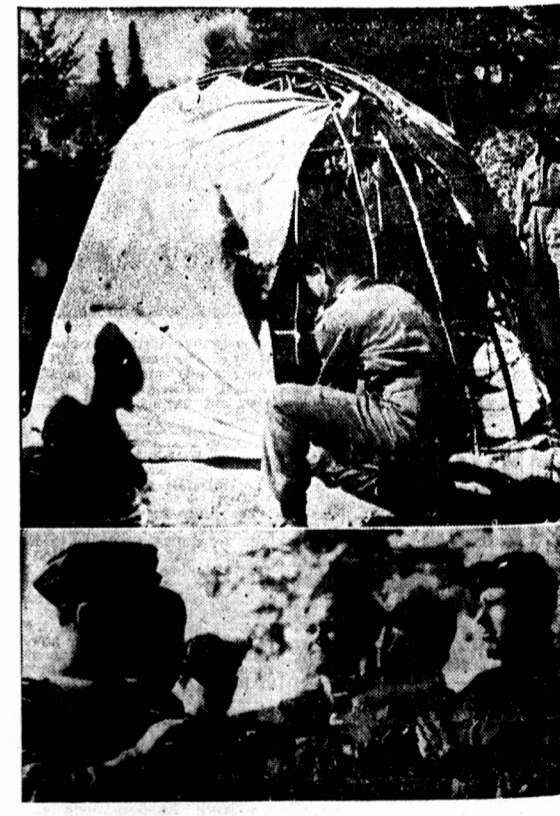
Protection from storms, or living quarters for men, can be built when the army fights in wooded terrain. This wigwam as at top is built by pushing birch saplings into the earth, then tying the bent tops together and covering the whole with canvas or tarpaulin. In the lower picture men at Venne Depot use the knife to make axe handles starting with a block of wood. Closeup shows how the knife is used by an expert. These men will be highly trained woodsmen as well as soldiers when they finish the Army's woodcraft course in the Quebec woods. (Canadian Army Photo.)
