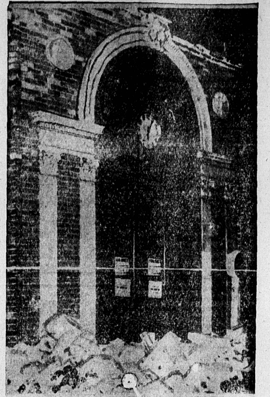
CLOCK STOPPED BY EARTHQUAKE SHOCK A series of earthquake shocks terrorized southern California March 10 and 11 when millions of dollars of damage was done, over one hundred people killed and thousands injured in Long Beach, Los Angeles, and other communities. Above is shown a clock which was stopped by one of the shocks as brick work of the building tumbled round about it.
