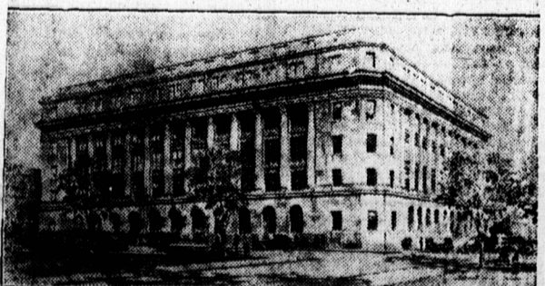
A house in which lived the Honorable Alexander MacKenzie, prime minister of Canada between 1874 and 1878 was torn down with several others to make way for a fine new home of the Metropolitan Life Insurance Company in Ottawa. It is to be ready for business by next autumn.
