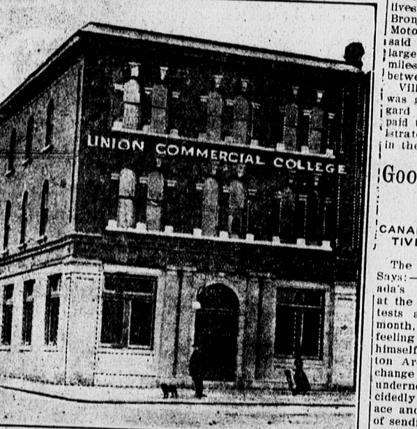
HOME OF THE UNION COMMERCIAL COLLEGE, ROYAL BANK BUILDING
