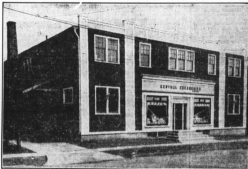
Central Creameries Office and Plant, Charlottetown
