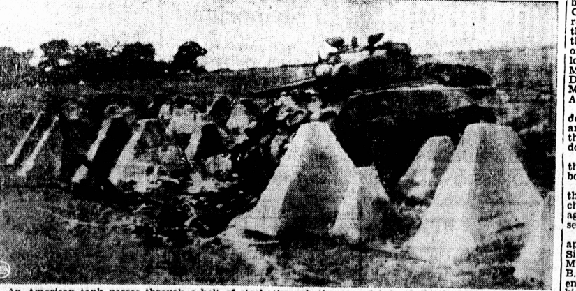
An American tank passes through a belt of steel and concrete dragons' teeth obstacles in the Siegfried Line, near Aachen, Germany, after Army engineers blasted a path. American troops pushed through the second belt of the fortifications. (Photo by NSA-Acme photographer Andrew Lopez for the War Picture Pool).
