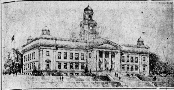
ADMINISTRATION BUILDING, ACADIA UNIVERSITY, WOLFVILLE, N. S.
