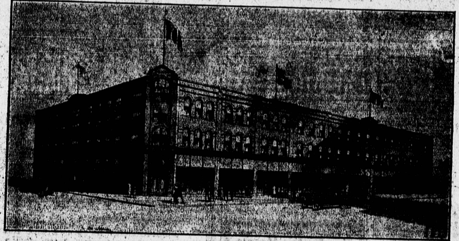
This entire block, with fifteen warehouses, comprises the Summerside plant of R. T. Holman, Limited.
