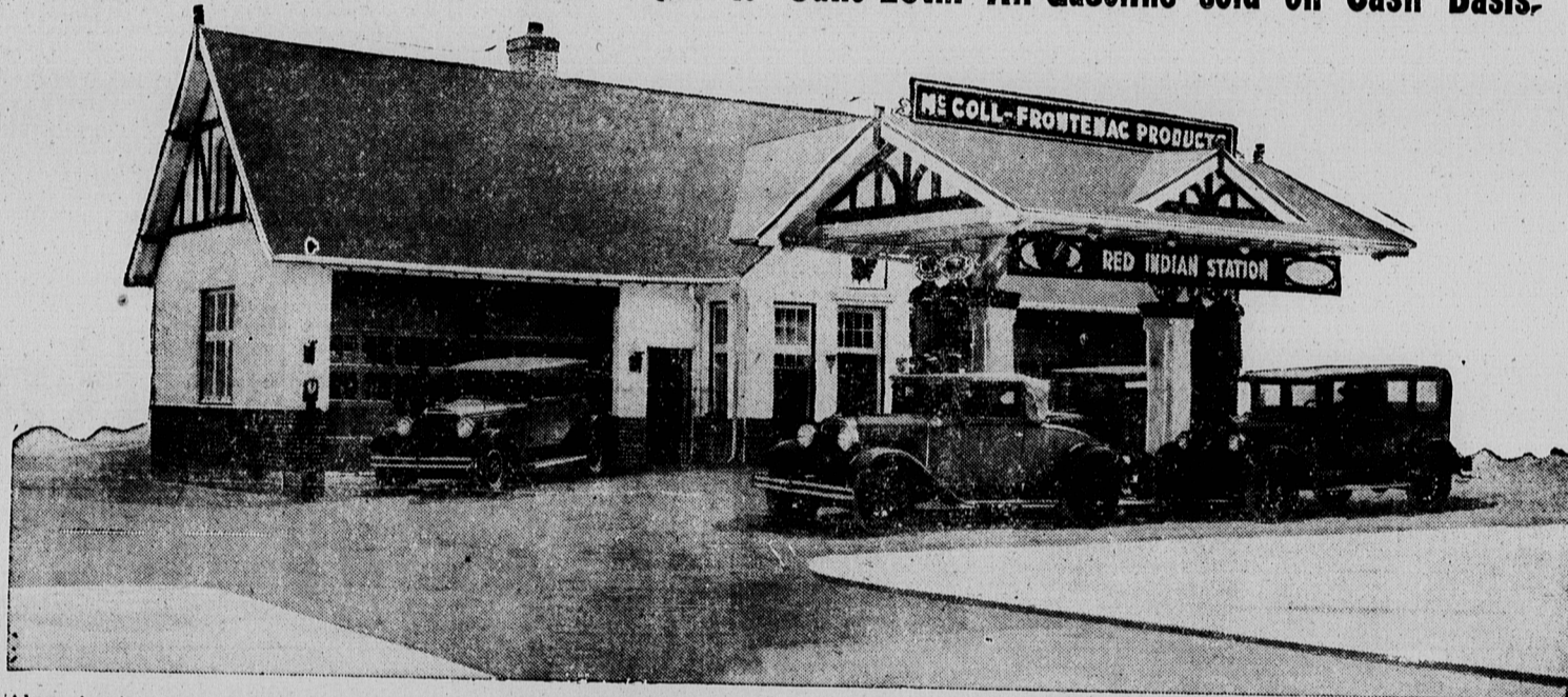
Above is pictured a typical McColl-Frontenac RED INDIAN Service Station. Stations of this type now dot the principal highways of the Dominion. In Summerside one has been opened on the corner of East Water and Eustane Streets, and one on the corner of West Water and Second Streets.
