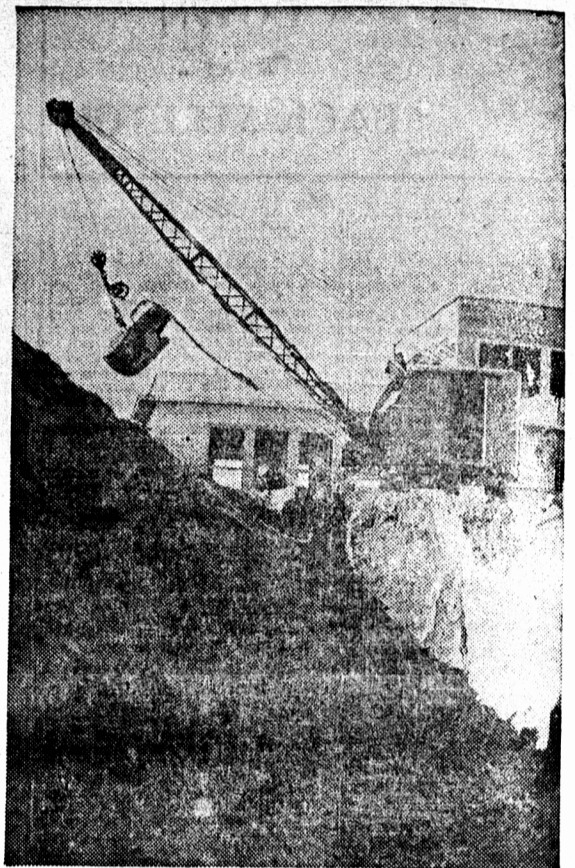
Construction work started the day after signing of the agreement. The Plan has not known a full day's holiday since. More than 140 aerodromes were built.
