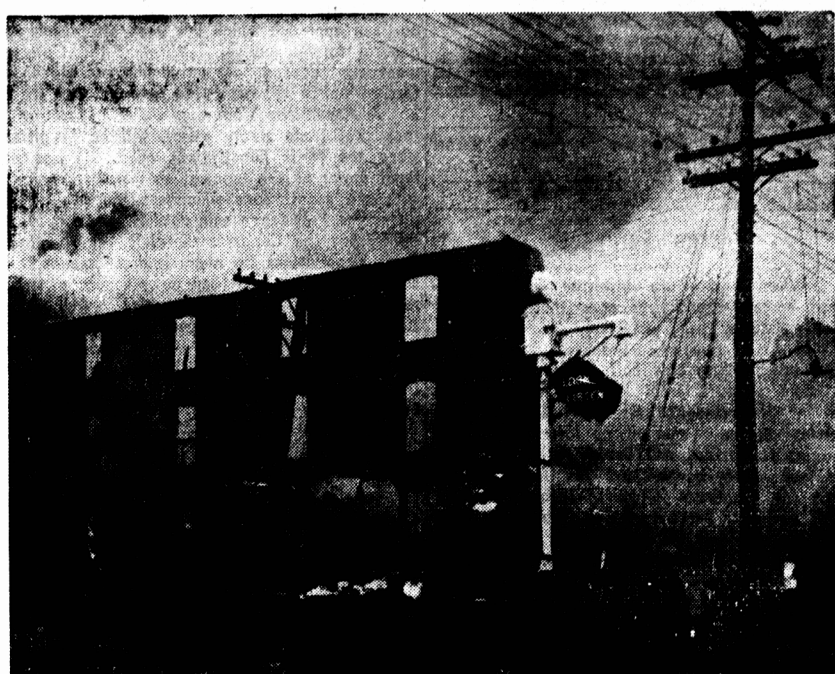
Gaunt brick wall standing after fire has completely demolished the older section of the Company's plant, with estimated loss of over half a million dollars.
