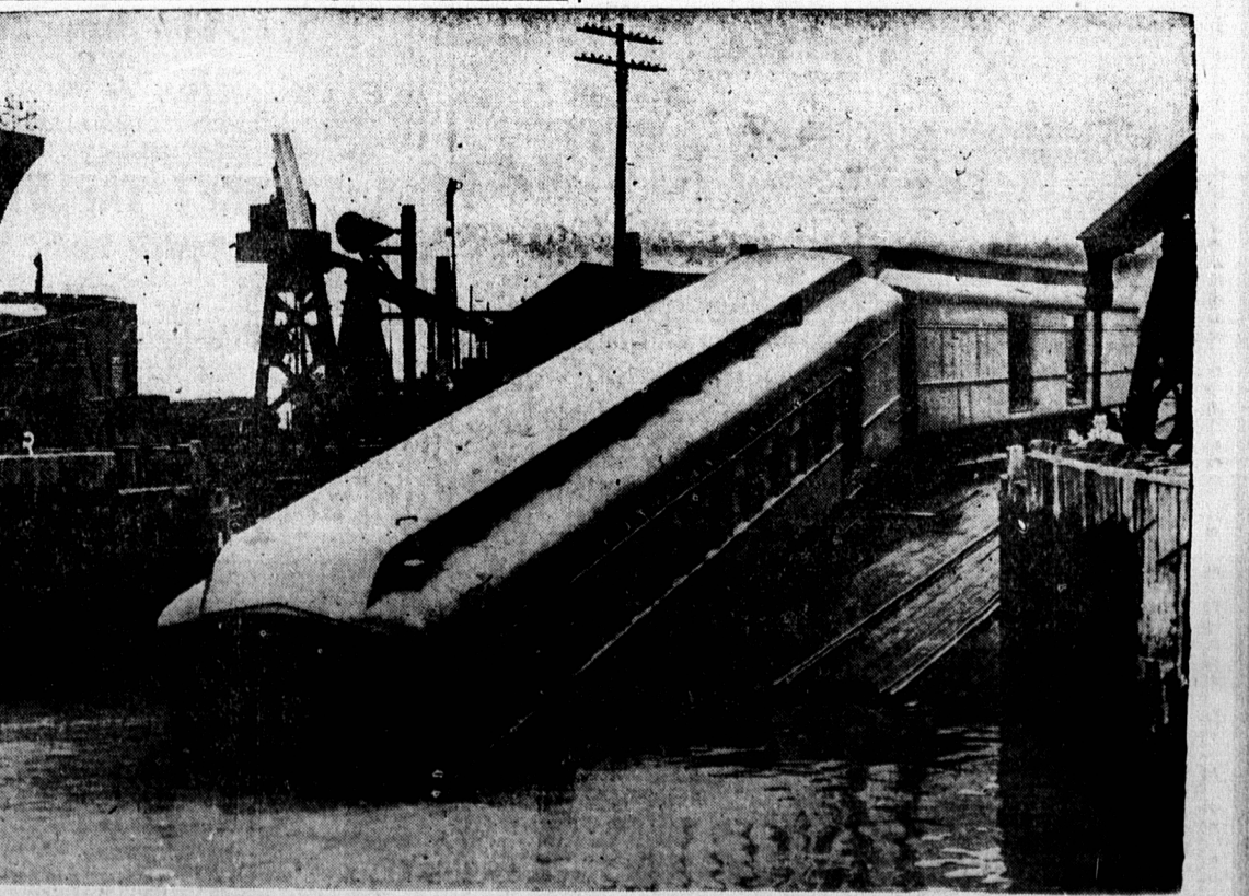
End of the line for this Canadian National Railway mail car was a surprise dip in the Detroit River at Windsor. When there was no rail block or car ferry at the track terminus, the train being shunted on the dock gave three mail men in the end car the surprise of their lives. They escaped from the partly submerged car by the rear door.
