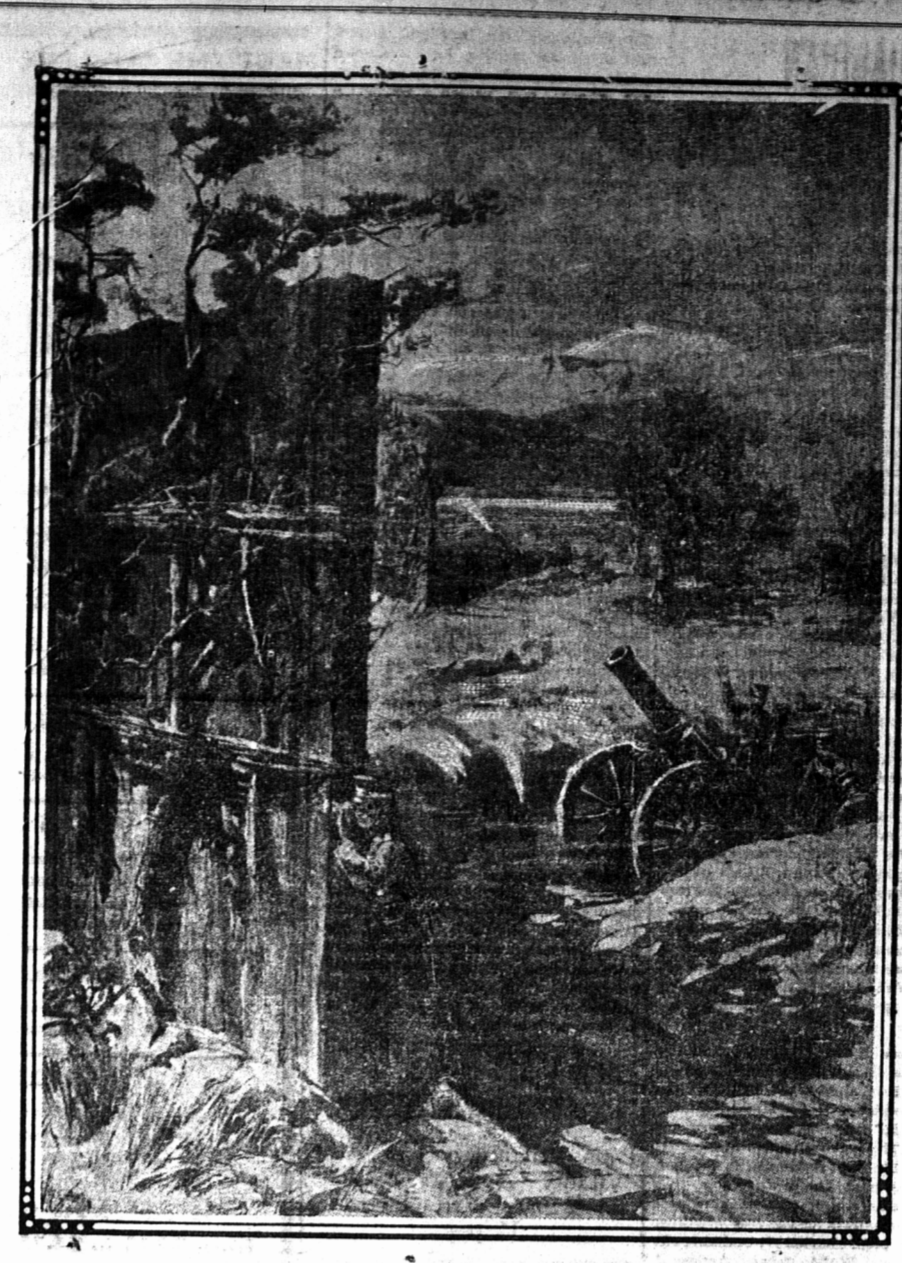
JAPANESE GUN-SHIELDS IN PLACE OF EARTHWORKS. This illustration is the best photograph that has so far gotten through the Japanese lines uncensored. It shows graphically the marvelous inventive ingenuity of the Japanese. These shields, which are made of timbers two feet thick and twenty-five feet in height, were erected by the Jap engineering corps by previous direction, and when the time came for the artillery to take their assigned positions and they had been located by the Russian batteries, the gunners were thoroughly protected from any scattering fire or stray pieces of shells.
