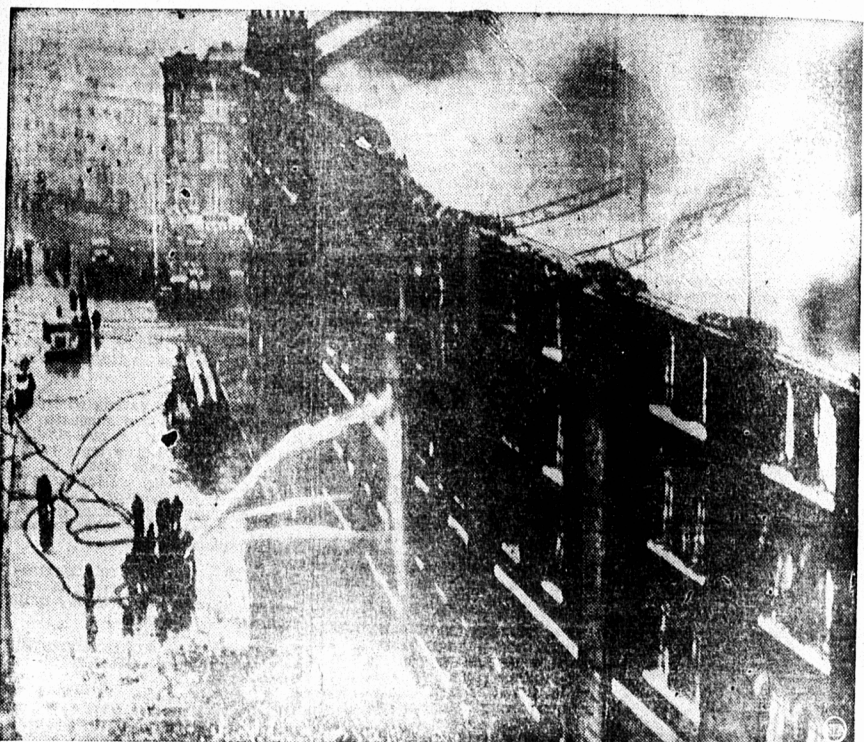
London's firemen vainly pour seemingly-puny streams of water against the raging inferno that left one of the capital's dock warehouses but a hollow shell behind a tall brick facade. Roaring blaze was started when Nazis, taking advantage of full moon, poured tons of bombs on the British capital in worst air raid of the war.
