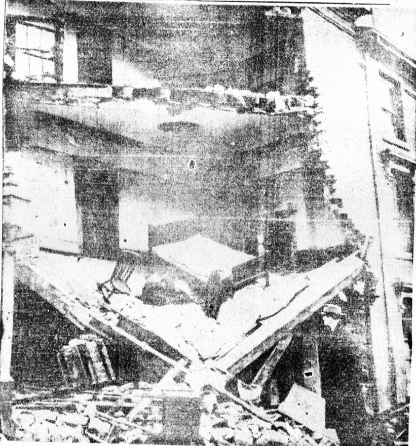
The wall is ripped away and the floor tilts at a crazy angle, but the bed is still in place in this Midland home after the passing of a Nazi bomber.
