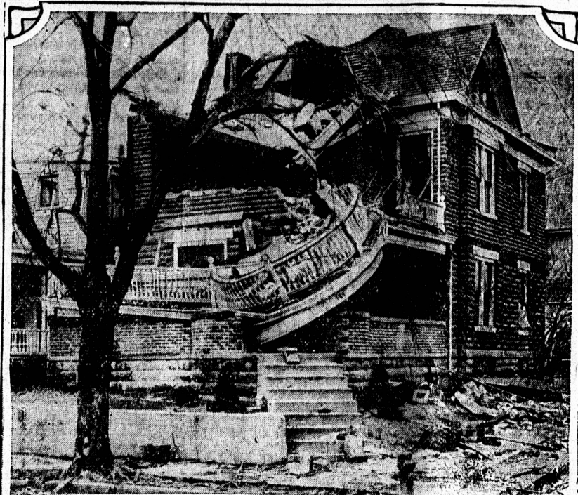
DAMAGE WROUGHT BY OHIO TORNADO
