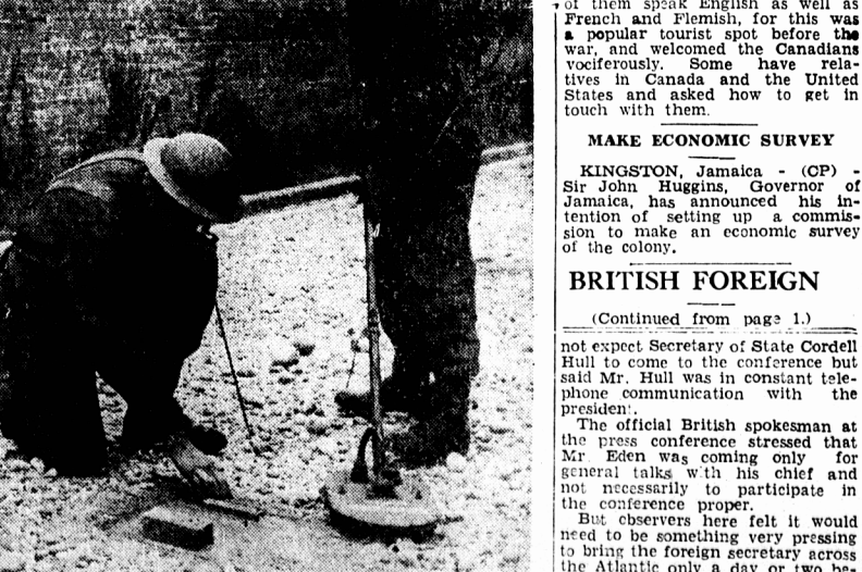
The Nazis in their headlong retreat from northeastern France had little time to plant mines or booby traps to slow the Allied advance. But Royal Canadian Engineers took no chances and here they locate a box mine on the road to Falls, near Dieppe. The mine detectors are Pte. J. Lafferty, Saint John, N. B., and Pte. C. A. Shaw, Arthur, Ont. (Canadian Army Overseas Photo).
