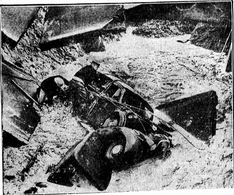
Boiling flood waters swept the foundations out from under this bridge at Del Mar, California, when the worst rainstorm in years deluged the state recently. The two automobiles were crossing when the bridge floor collapsed into the swollen stream. Scores of automobiles were stranded in as many towns and villages during the $25,000,000 flood, which resulted in death for more than 100 persons. So turbulent was this flood stream that salvaging operations were long impossible.
