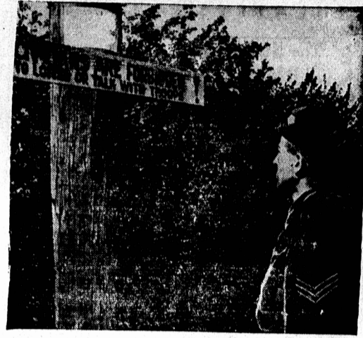
Invasion preparations in Great Britain, many of which will not be fully disclosed until Germany's final submission, included the widening of British highways and the strengthening of many bridge spans to carry heavy invasion equipment. In concentrated areas, signs, as shown here, warned civilians not to talk with soldiers.
