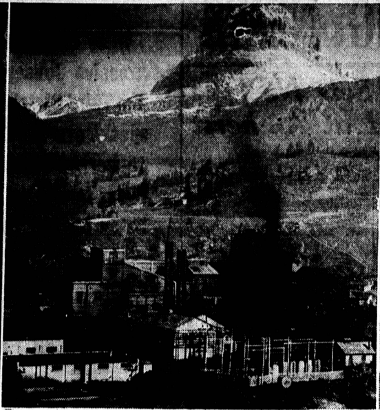
Western miners work with the majestic Rockies as a background. Above, black smoke of coal preparation plants at Coleman, Alberta, rise to the clear sky.
