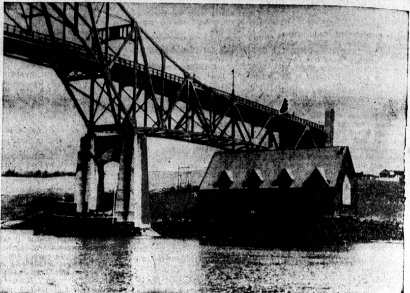
This sea-going church, being transported by barge from Hull to Buzzards Bay, Mass., is on the last leg of its journey through Cape Cod Canal as it passes under the Sagamore Bridge at Bourne. Unused in Hull, the church is now the property of the parish of St. Peter-on-the-Canal Episcopal Church, whose congregation will turn out to greet their new building when it docks.
