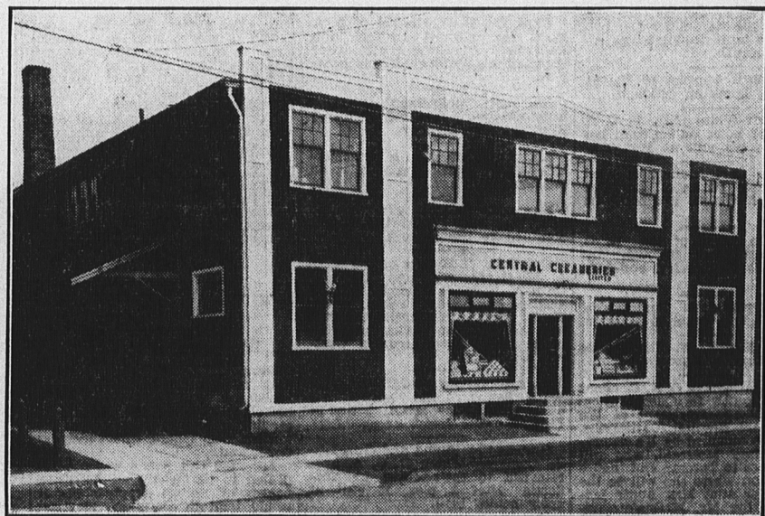
Central Creameries Office and Plant, Charlottetown
