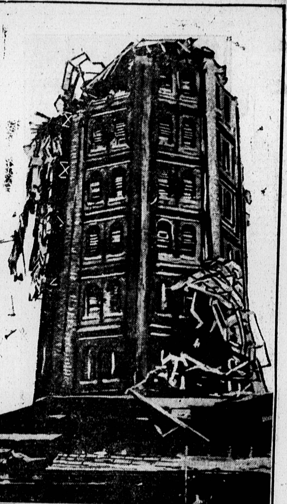
One of the first photographs showing the result of earthquakes in Japan to reach the American Continent. This was taken on the day following the initial shock by one of the refugees who was a passenger on the Canadian Pacific S. S. "Empress of Australia," which performed such a heroic part in the rescue of the sufferers; and it shows how a thirteen-story building crashed from the seventh floor into the street Wilson Howatt, which occurred in
