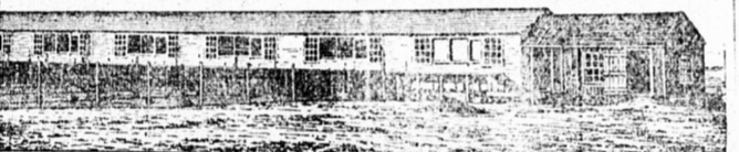
The latest curtain front poultry house.
