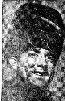
Eugene Morasse is a welder one of hundreds on the job.
