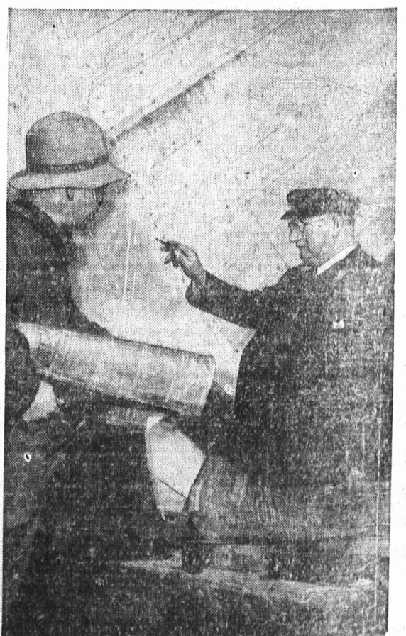
The double-planked stem, soon to crash through ocean swells is checked by a shipyard foreman. Craftsmen like these are foundation of the Royal Canadian Navy.
