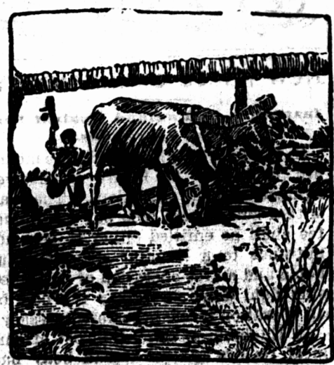
IRRIGATION PUMPING WORKS.
