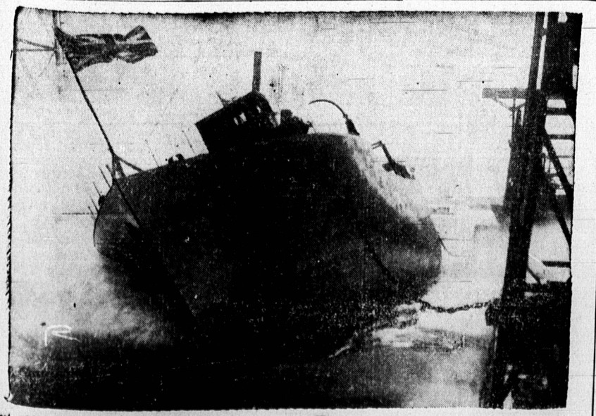
Latest addition to Canada's navy, this sleek sub-chaser took to the water gracefully in a broadside launching at a Georgian bay port recently. The pull of the launching plunger snapped a heavy check-rope holding the bow to the t. Getting off to a flying start, the corveta beat the christening bottle in the first attempt. The ceremony was completed) with smashing of the champagne bottle as the craft made the launching waves in the slip.
