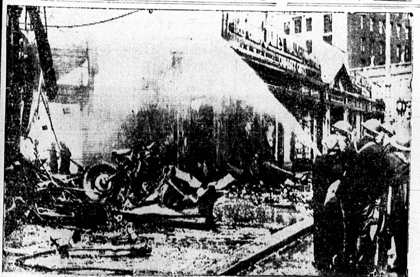
One of the 185 German warplanes shot down in mass raids on London, Sept. 15, this big Dornier bomber crashed on the roof of a jeweller's shop across from Victoria station, where air raid workers are pouring water on its blazing wreckage. The plane fell apart as it came down, and odd parts were scattered over a wide area. Londoners saw dozens of raiders fall as R.A.F. fighters piled up their biggest score of victories to date. Germany lost 450 airmen in the day's raids.
