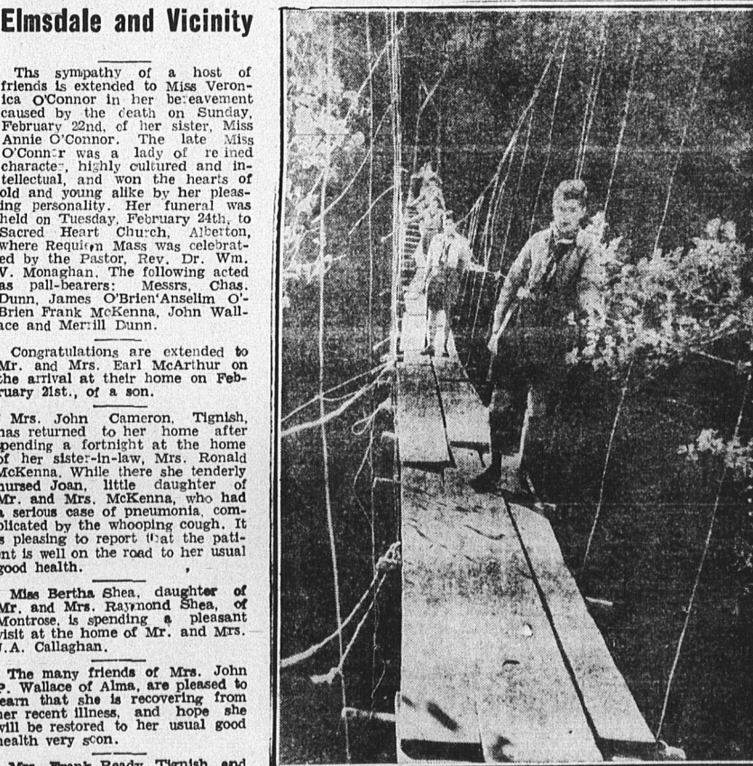
A Scout-built bridge. To save a three-mile walk, following an evacuation, Boy Scouts of Tisbury School, on the river Wye, near Monmouth, England, built this 167-foot suspension bridge. They did the entire work, felling trees, squaring them, and doing the knotting and lashing.
