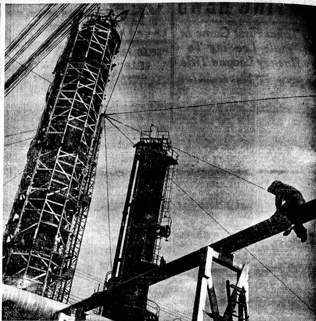
Giant tower at Sarnia synthetic rubber plant took five days to move on three flat cars from Montreal, was one of the biggest jobs in building Polymer plant.
