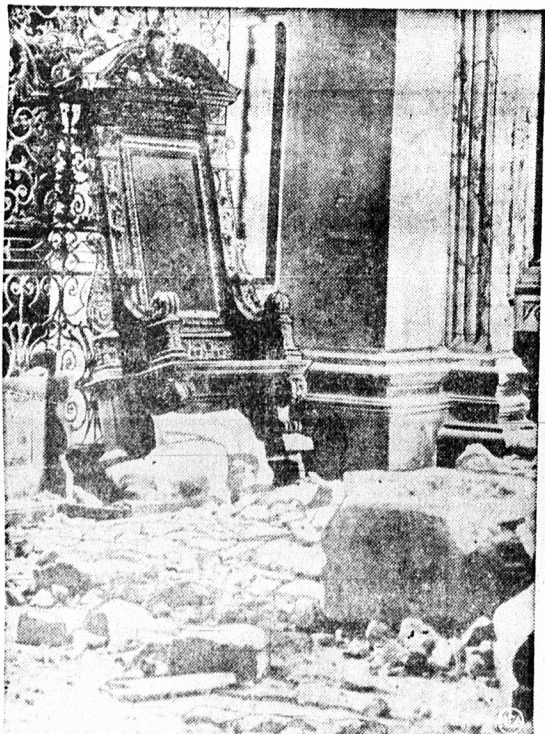
Tipped back against an iron grille, the Bishop of London's throne stands amid the wreckage of the high altar in St. Paul's Cathedral. Damage was done when Nazi bomb, exploding on hitting roof, toppled great chunks of masonry on the shrine, 90 feet below.
