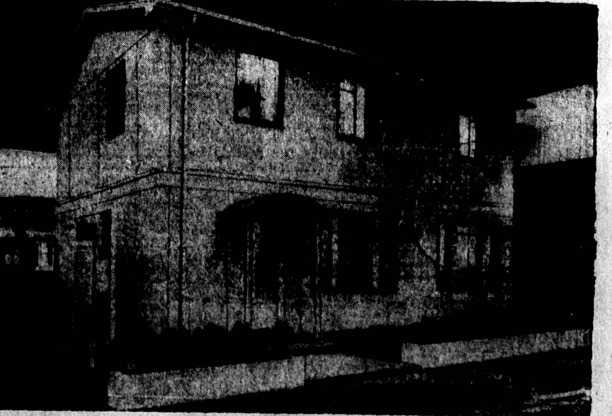
Featured exhibit at London's Ideal Home Exhibition is this two-story pre-fabricated aluminum house. It can be assembled on a site in one day. Ground floor sections are built complete in every detail, including equipment, so that site work is limited to bolting them together.
