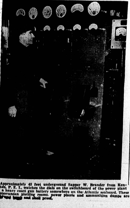
Approximately 45 feet underground Sapper W. Brander from Kennington, P. E. I., watches the dials on the switchboard of the power plant for a heavy coast gun battery somewhere on the Atlantic seaboard. These subterranean plotting rooms, power plants and ammunition dumps are well protected and well guarded.
