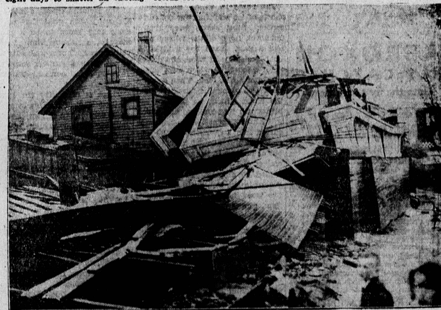
MANY BUILDINGS DESTROYED BY OHIO STORM
