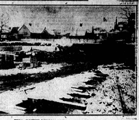
THE FOUNDATIONS OF THE NEW C. N. R. HOTEL
