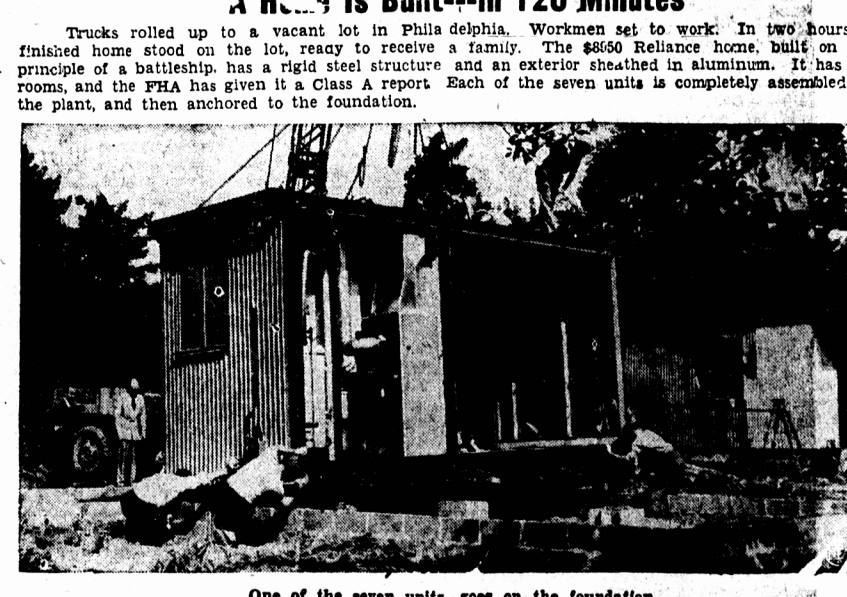
One of the seven units goes on the foundation.
