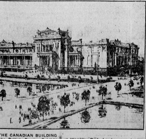
THE CANADIAN BUILDING. As it will look when completed at the British Empire Exhibition at Wembley Park, London next April.
