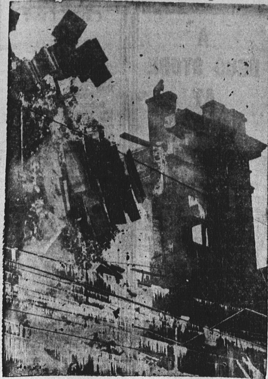
After a two-hour battering from high-pressure hose proved ineffectual, firemen pulled down the shaky walls of the Imperial Bank building, which burned in Toronto. This photo shows tons of masonry tumbling to the streets. Firemen used ladders to fasten long ropes to protruding beams and then pulled. Brick and stone came tumbling down with a thundering roar. The fire raged more than 17 hours. Damage was placed at $110,000. Telephone wires were sheathed in ice from tons of water poured into the building.
