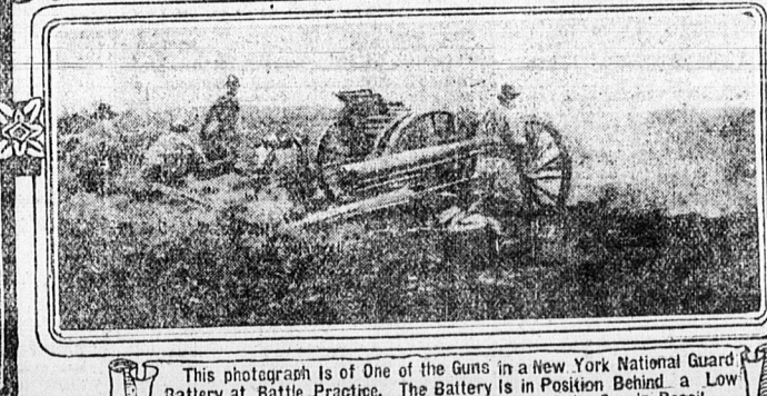
This photograph is of one of the guns in a New York National Guard Battery at Battle Practice. The Battery is in Position Behind a Low Ridge, Completely Masked. Note the Barrel of the Gun in Recoil, Thrown Back on the Carriage.
