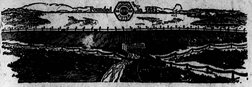
The largest earth dam in the world, on the Saluda River near Columbia, South Carolina, as it will appear when completed
