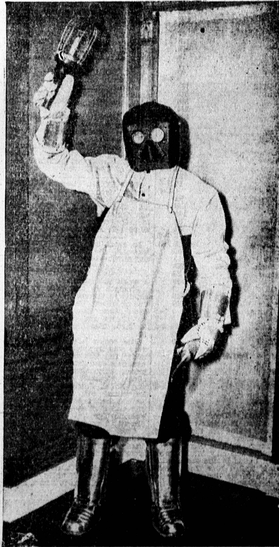
This is neither a modern Diogenes looking for a honest man nor a visitor from Mars equipped for a bit of interplanetary war. It is a "manquin" demonstrating what the prudent workers wears in many modern factories. The helmet protects the head from flying metal fragments. The asbestos gloves are steel reinforced to prevent burns and bruises. The safety lamp guards against shocks. The glittering boots are for more than ornament. They keep the wearer's toes from being crushed if he drops something heavy. This Costume of Gadgets was demonstrated at a Pittsburgh safety meeting a few days ago.
