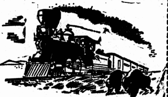
TRADE Across the prairies... over the Rockies... on to the western sea roared the iron horse... builder of trade... bringer of progress and prosperity.
