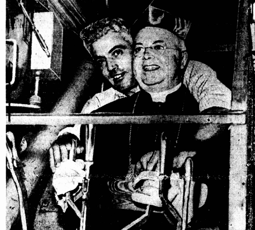
With a Cardinal at the controls, this huge power shovel is preparing way for construction of new $750,000 De La Salle college, "Oaklands", in Toronto. His Eminence James Cardinal McGaughey attended ceremonies marking start on new Roman Catholic high school and is seen here sharing with help of operator, J. Famiglietti.
